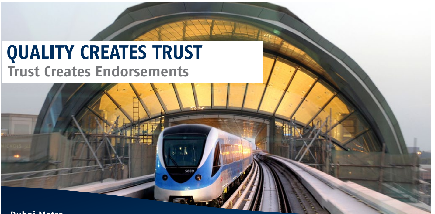
Dubai Metro United Arab Emirates
